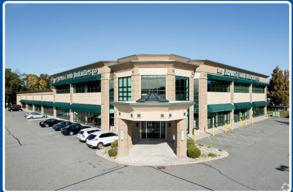
Building prior to new construction
